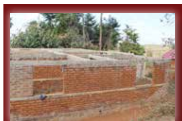
Maanda's family house under construction in Singu village
