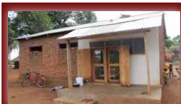
Shida's family house in Manungu village
